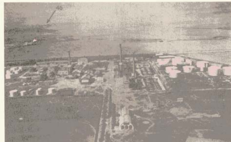
PHOTO E... (1929), looking W TARGET 40 - Concordia Vega Oil Refinery. TARGET 46 - (in distance) Redeventza Refinery.
