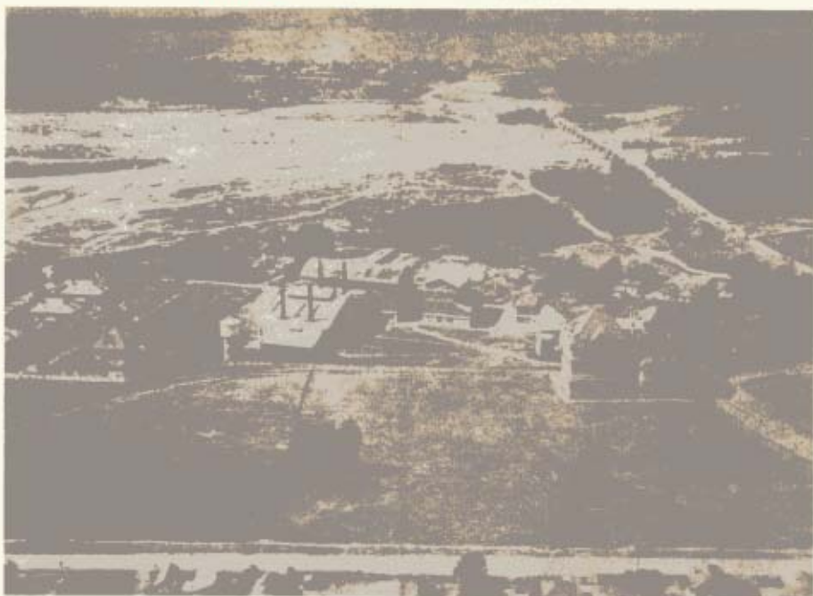
PHOTO K...FLORESTI (1929), looking W. TARGET 80 - Floresti Electric Power Station.
